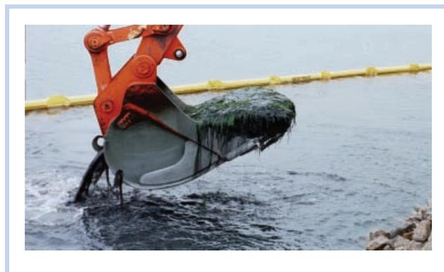
**Figure 4.** Dredging operations impact to habitat. Dredging shown removing contaminated sediment and eel grass communities. (Source: Kimberlee Keckler, USEPA.)
